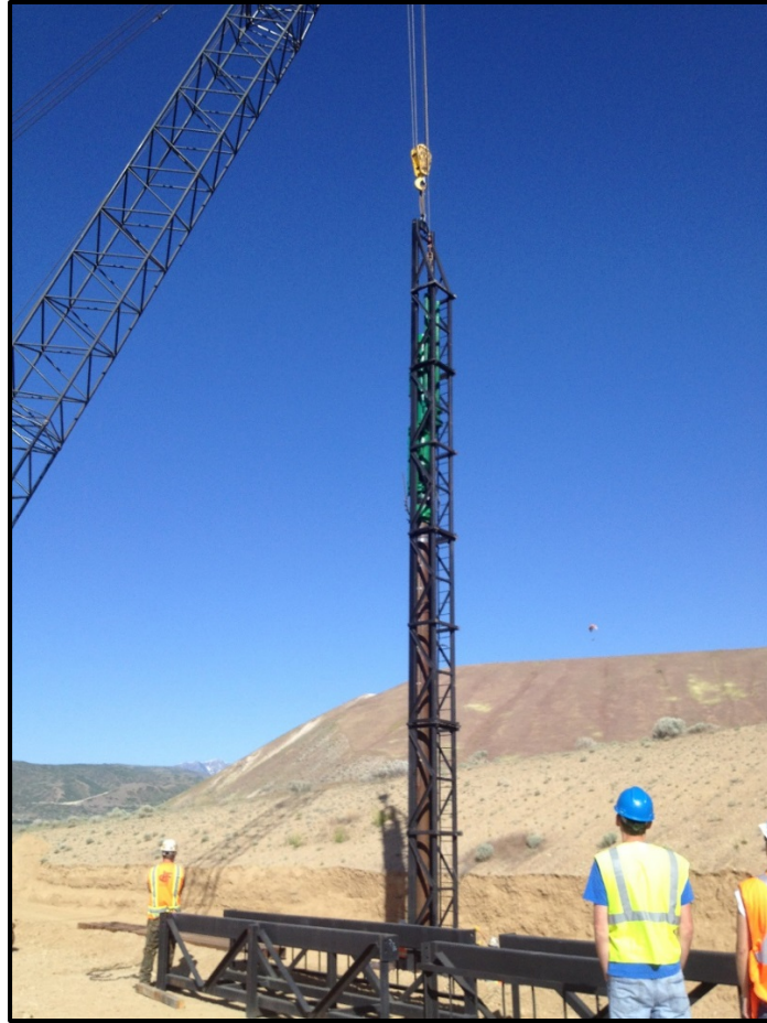
Figure 3-3: Installation of piles using a diesel hammer.
