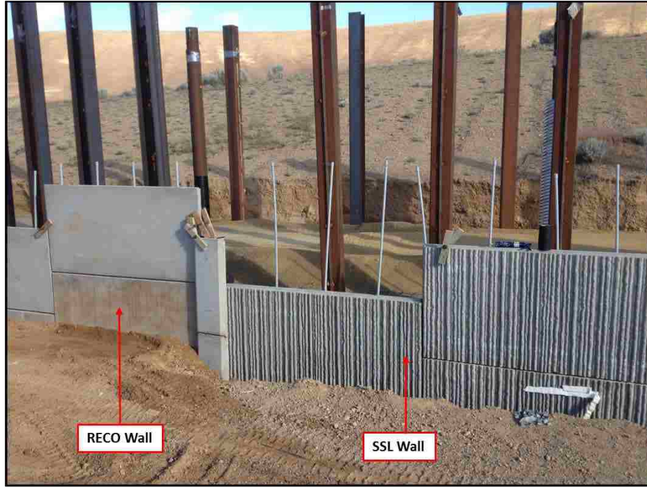
Figure 3-7: Different wall systems used for this project.
