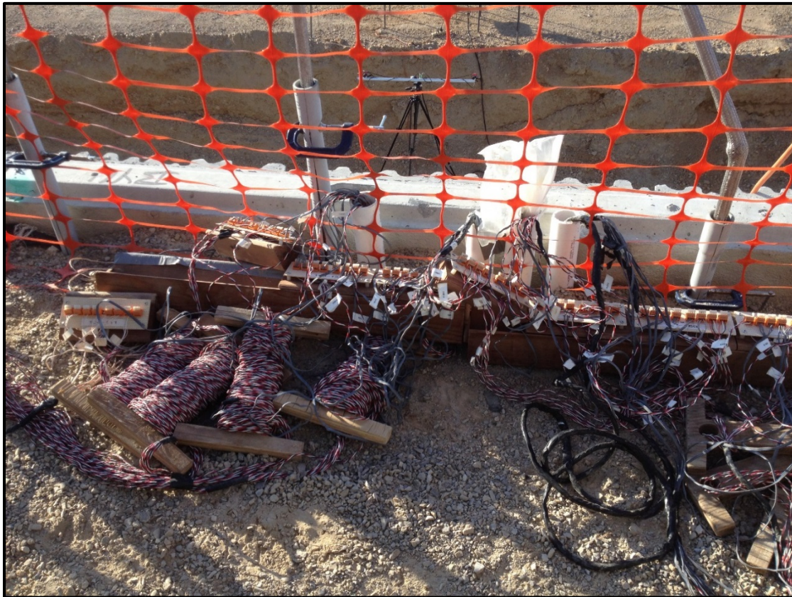
Figure 4-4: Strain gauge connections to terminal strips.
