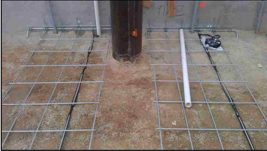
Figure 4-3: Typical strain gauge setup for a welded-wire grid layer.
