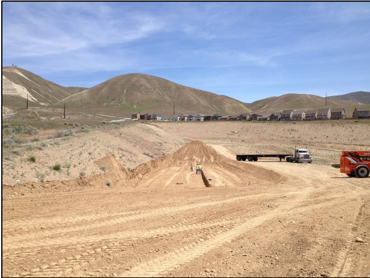
Figure 3-2: Project site after completion of site grading.
