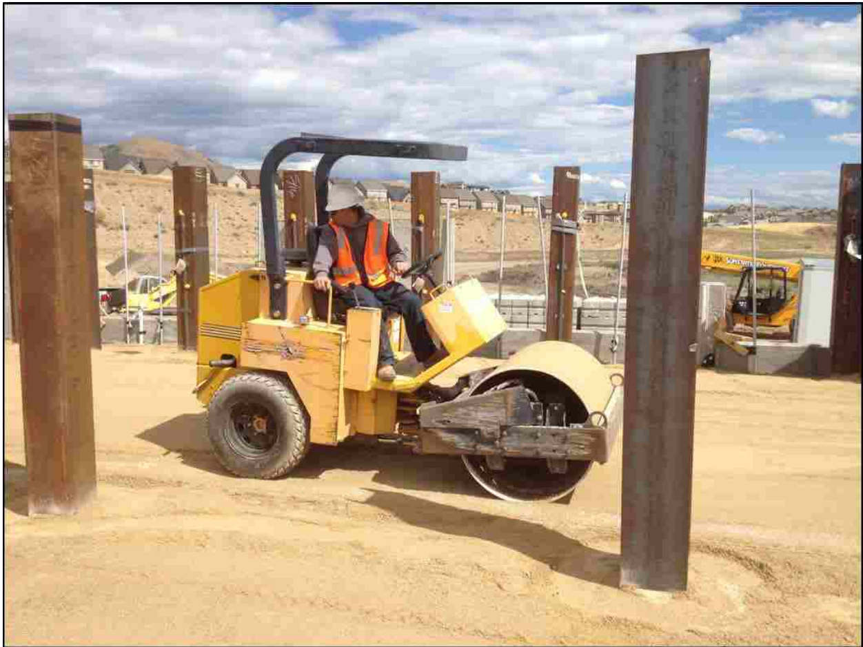
Figure 3-12: Compaction of backfill behind the test piles using a vibratory roller compactor.
